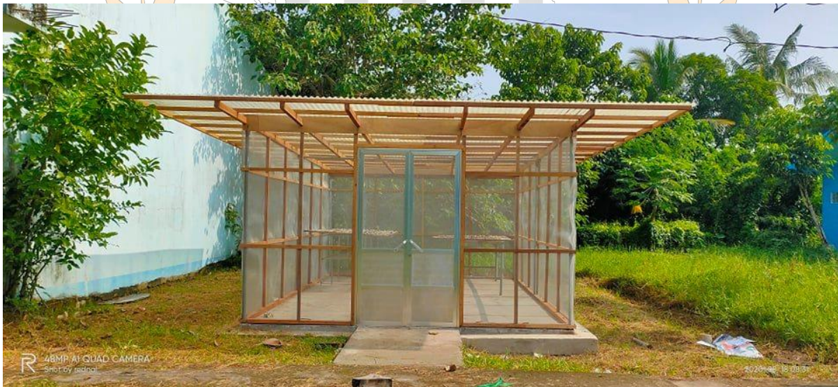
Figure 1: The upgraded fish solar dryer
